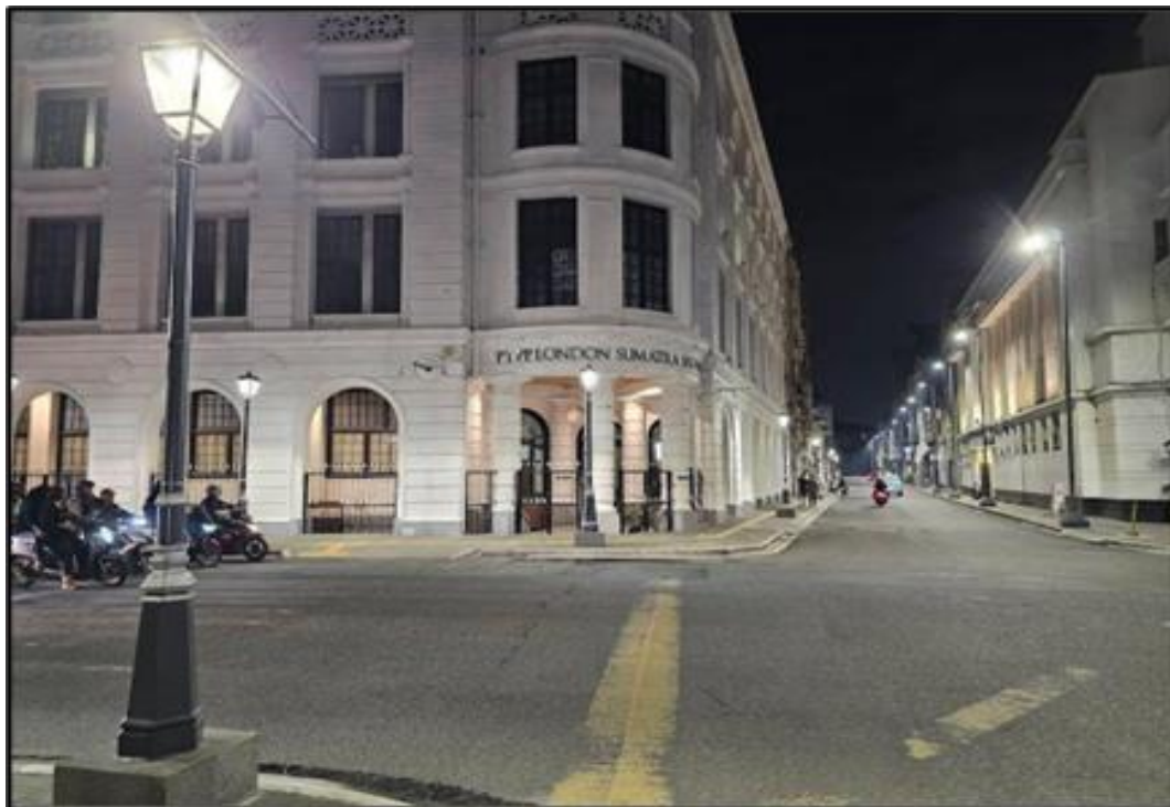
Figure 4. Lonsum Building at night
