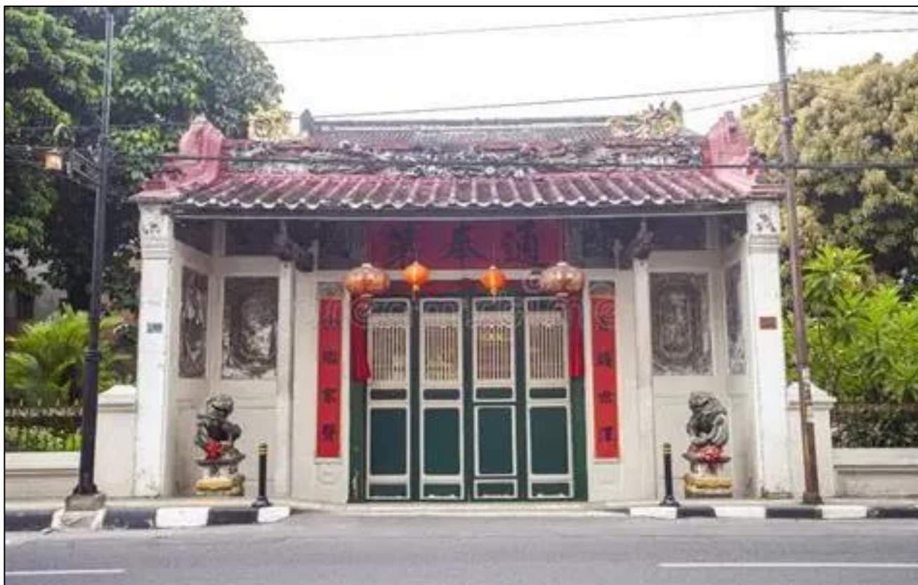
Figure 5. Tjong A Fie Building from Outside
