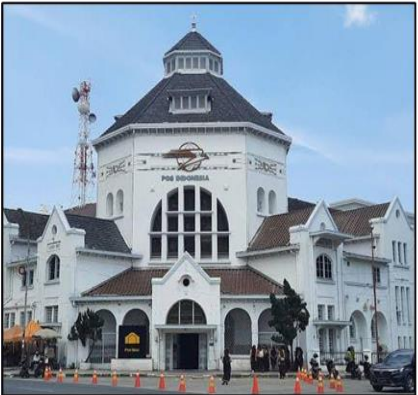
Figure 7. Pos Bloc Building from Outside
